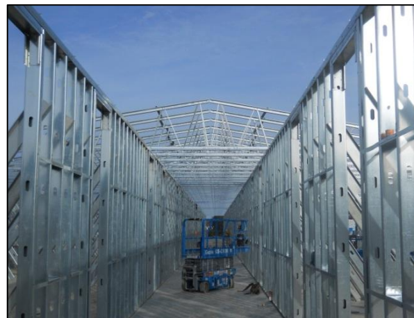
Figure 2: Metal Stud Bearing Walls - Courtesy of Barton Malow
