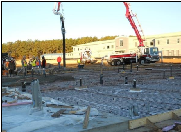
Figure 3: Slab on Grade - Courtesy of Barton Malow
