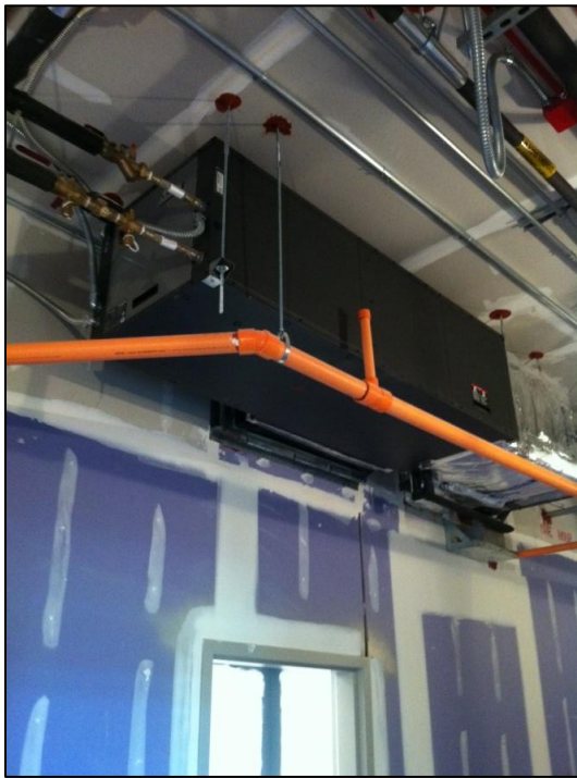
Figure 5: Heat Pump - Photo Taken by Kendall Mahan
